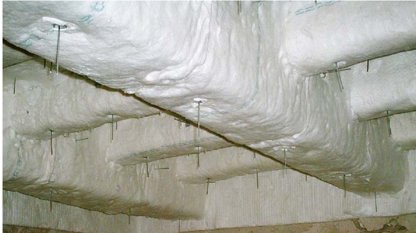
Typical deck installation around stiffeners
