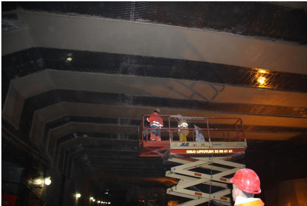
Photograph: FireBarrier 135 being applied by Innovative Fire Services in the Bjørvika Tunnel. The material is supplied as a powder and then mixed with water and sprayed into place using a standard cement spraying machine. Alternate sections are sprayed. The sections are formed by metal rails which also act as the installation thickness guide. These rails are then removed before the adjacent sections are sprayed.
