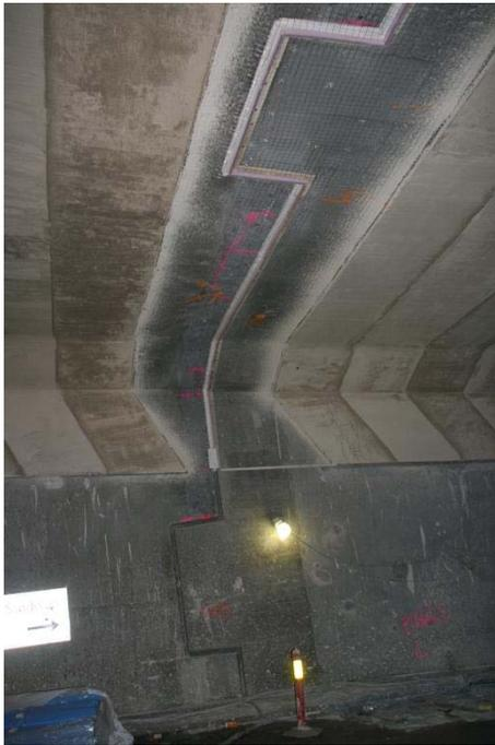
Photograph: Expansion joint sealing system installed shown before installation of the FireBarrier 135
