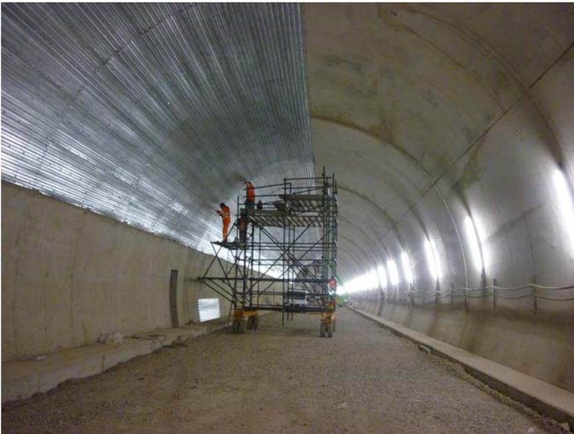
Fire protection of the wall is achieved using FireBarrier 135 which is spray-applied directly to the steel and additionally supported using steel wire mesh
